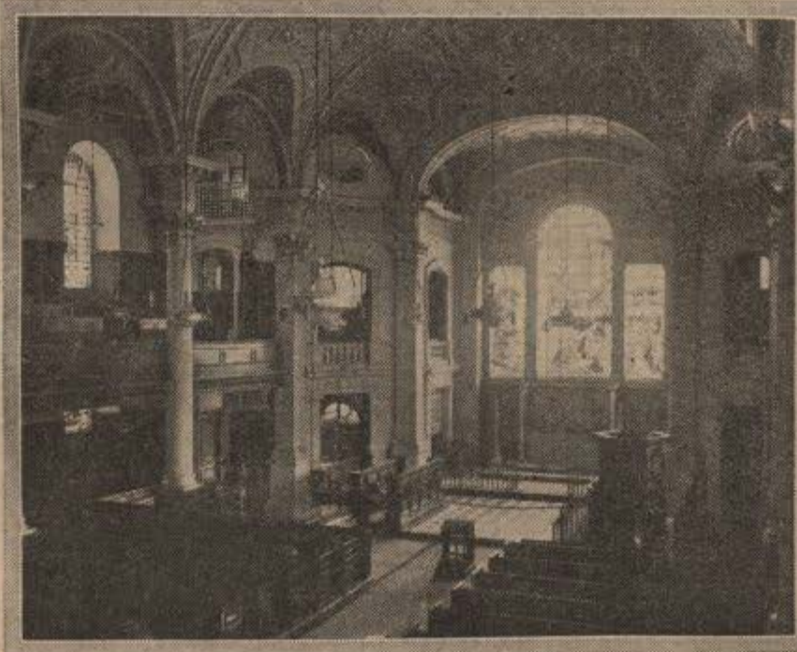
THE INTERIOR OF ST. MARTIN-IN-THE-FIELDS.
